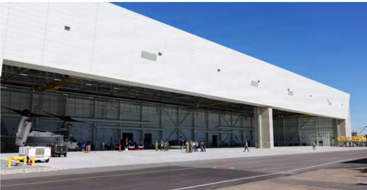
More than 80 FRCSW artisans, engineers and support personnel will work in the new hangar daily, using a layout they helped design to maximize efficiency and safety.
