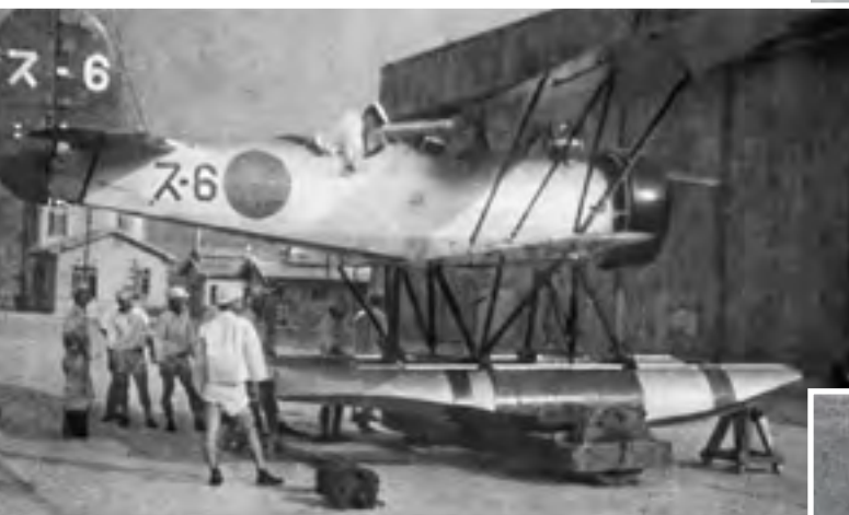
A production Watanabe E9W1 reconnaissance floatplane assigned to submarine I-6 undergoes a technical inspection at Kure Naval Base in 1937. Note the Japanese character and Roman numeral on the vertical tail.
