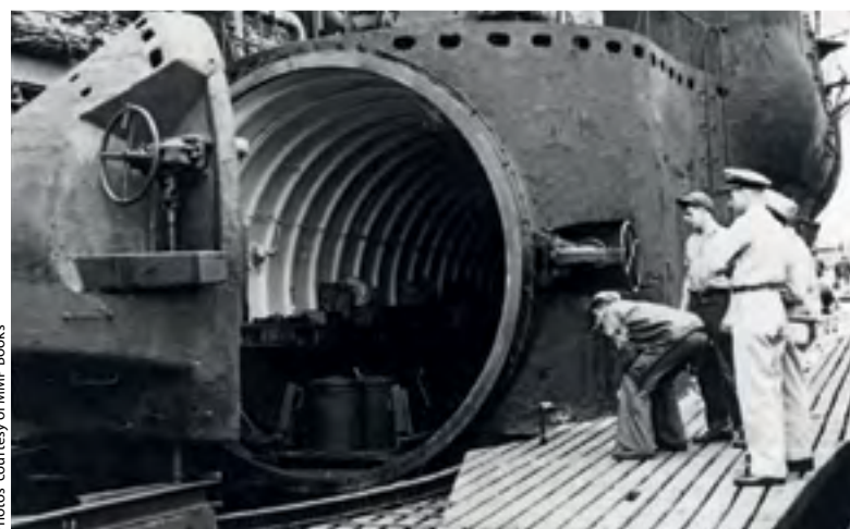
The watertight cylindrical hangar of the I-400 submarine, designed to house three folded Aichi M6A1 Seiran seaplanes.
