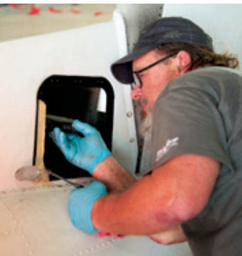
Thomas visually inspects his work to ensure proper bonding of the rib's faying surfaces. Heat lamps are placed on both sides of the aircraft to accelerate curing. Thomas uses a digital temperature laser gun to monitor the dorsal fin's skin temperature to ensure it doesn't exceed the recommended temperature.
