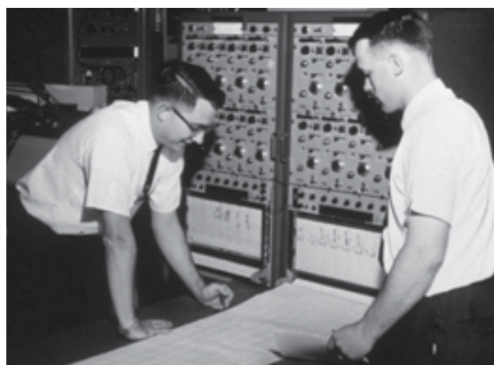
Strip charts were the test engineer's primary tool in the early 1960s during flight testing at the Naval Air Test Center at NAS Patuxent River, Md.
